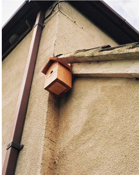
Birdcam positioned over the door into the utility room
